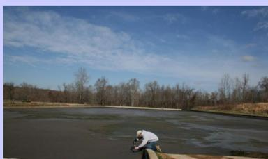
Sludge drying in a lagoon prior to land application.
